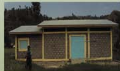
Grain Store Constructed (Kebele 09)
