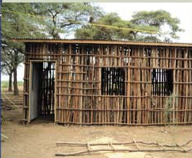
The house under construction.
